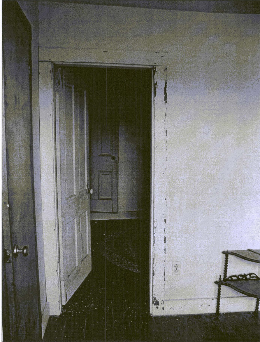
Figure 41. The partition wall divides the Period 4 space into two rooms.
