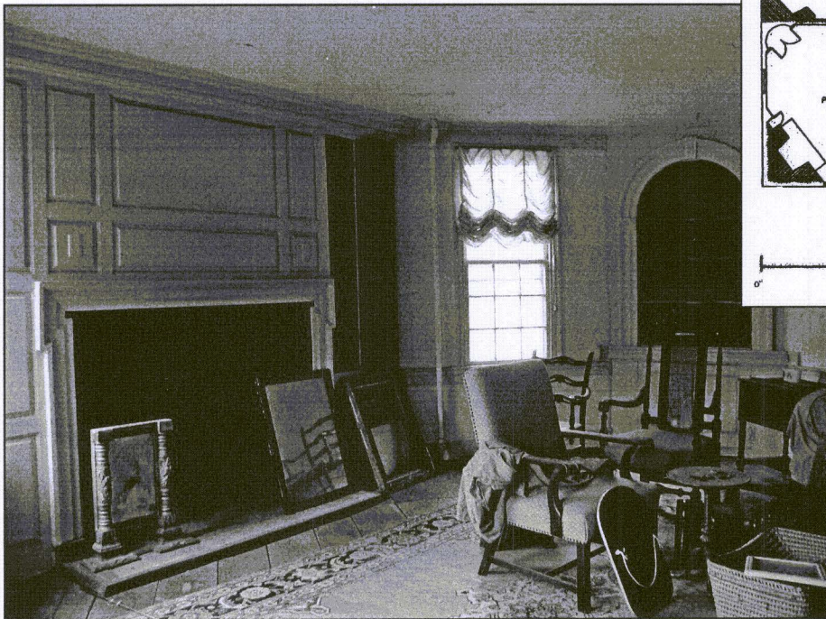
Figure 26. Period 1, first floor, south corner fireplace and west corner cupboard.
