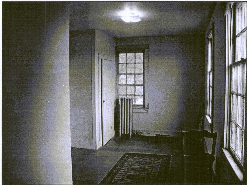
Figure 39. Period 4, second floor. Closet space (shown in the left of this photo) and a partition wall divide the Period 4 addition into two rooms.
