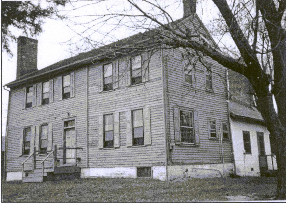
Figure 6. Perspective photo showing southeast and northeast elevations, circa 1998.
