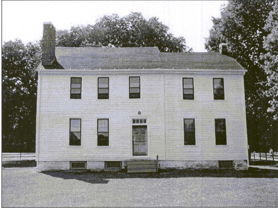
Figure 4. Southeast (front) elevation, summer 2002.
