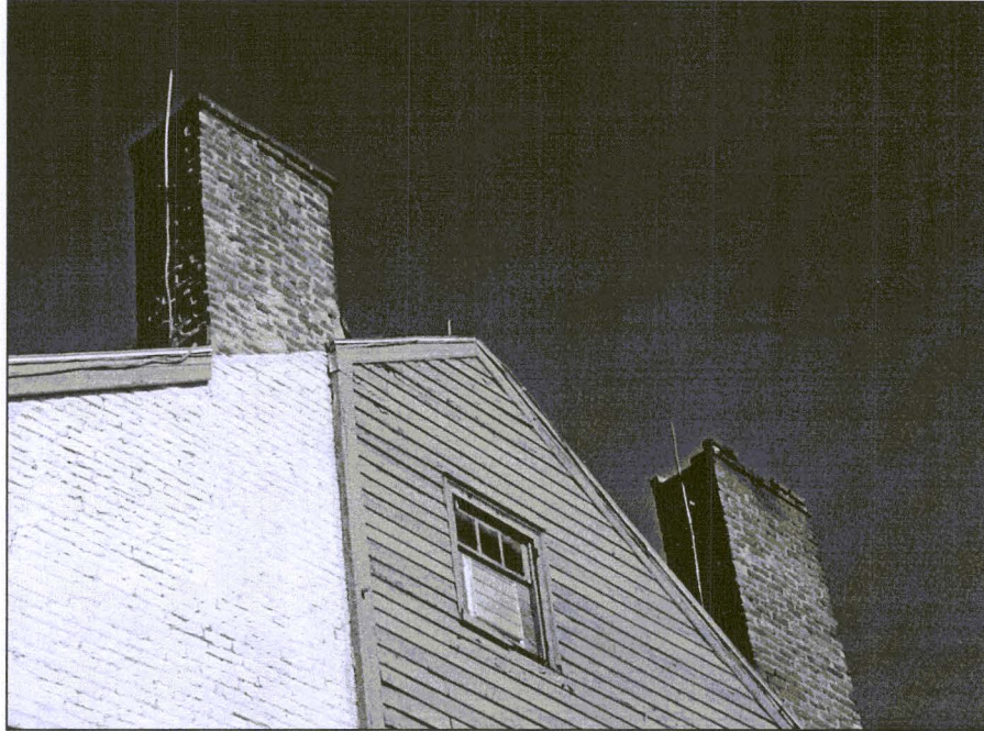
Figure 12. Detail of chimney stacks: Period 1 (right) and Period 2 (left), 2000.
