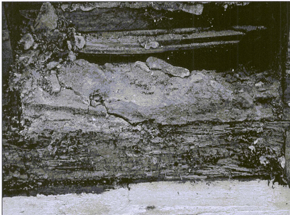
Figure 17. Detail of the sill plate, Period 4.
