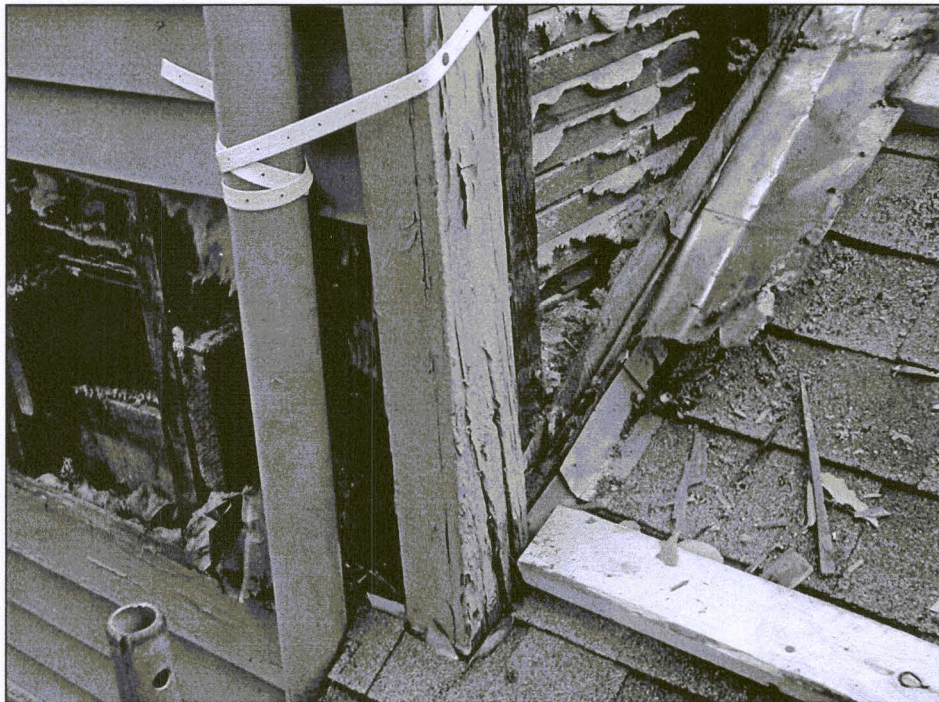
Figure 19. Clapboard to the left of the corner post was also removed.
