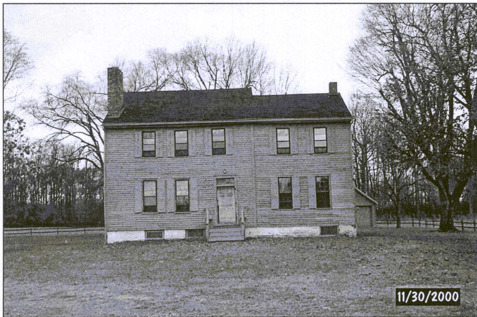
Figure 23. Front elevation of the Brecknock Manor House.
